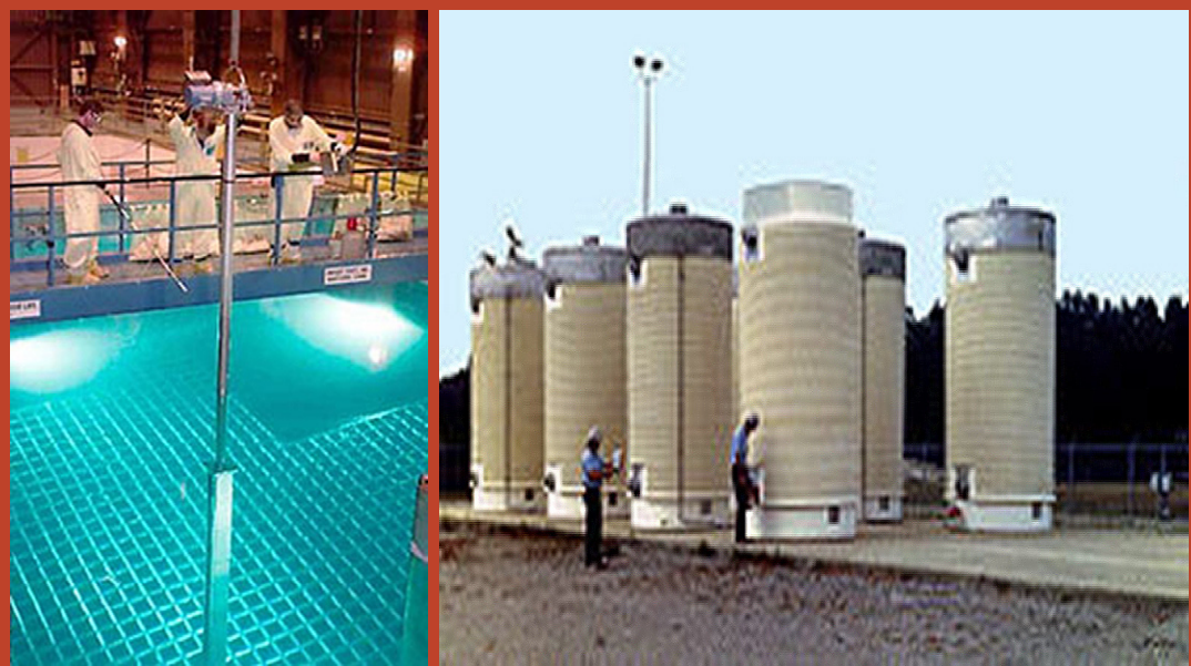
Figure 5. Spent fuel storage pool and dry storage area
